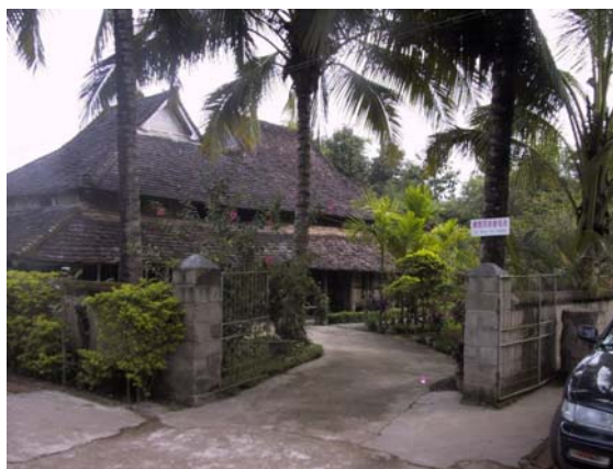
Figure 2.1 “Visiting Site of Dai Residential Building” Labelled on the Dai Home Visiting
