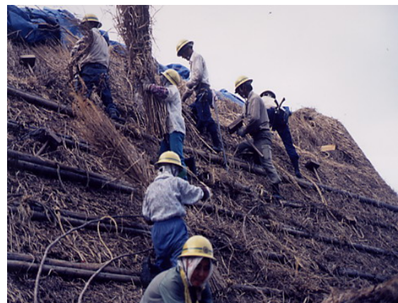
Figure 9.8 Repairing Thatched Roof of
